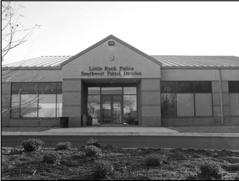
The Southwest Police Station off of Baseline Road is an excellent community resource.
